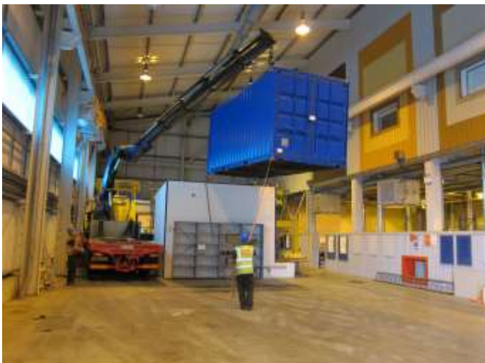
Figure 5.3: Installation of the shipping container for the storage vessels
