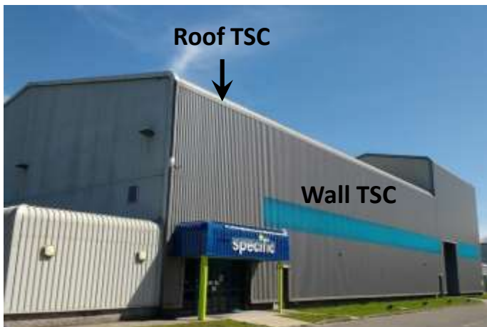
Figure 3.2: Southwest elevation showing Roof and Wall TSCs
