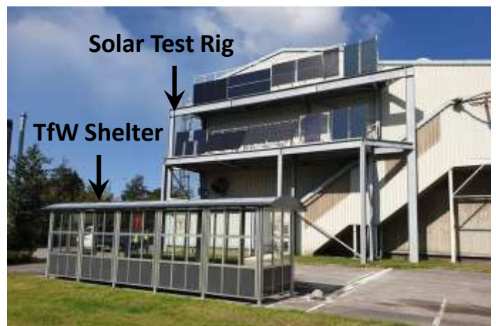
Figure 3.3: Southeast elevation showing Demo Rig and TfW Shelter
