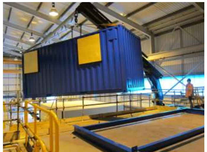
Figure 5.4: Installation of the shipping container for the storage vessels
