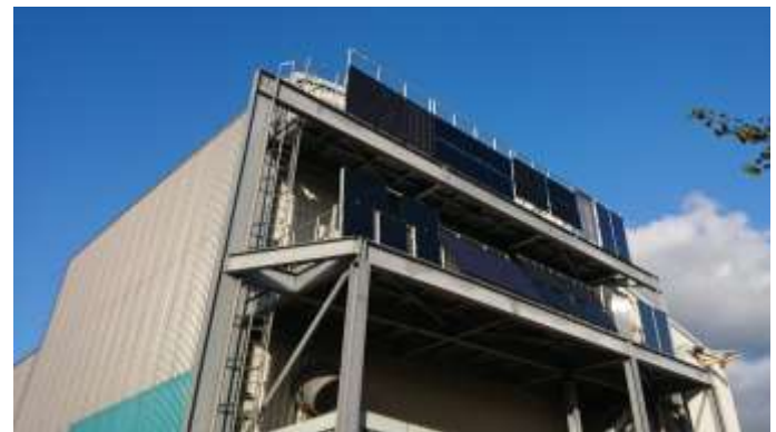
Figure 7.2: The Solar Test Rig – Close up
