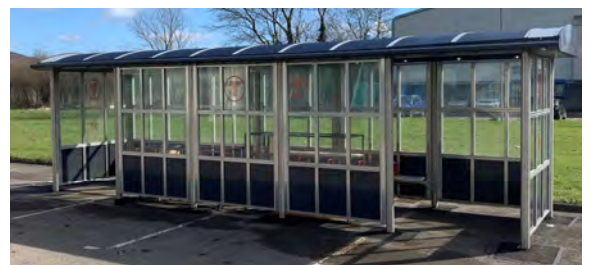
Figure 3.2: BIPV on a curved rail shelter roof
