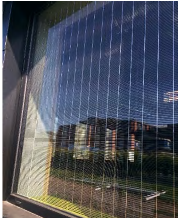
Figure 3.5: Pilkington Sunplus™ BIPV window
