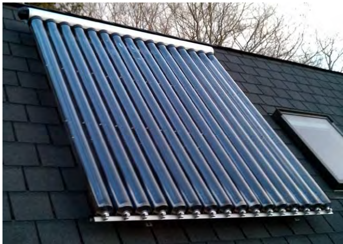
Figure 4.1: Photograph of an Evacuated Tube Solar Thermal Collector
