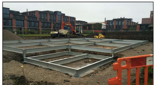
Figure 17: The steel screw pile foundations and the steel grid to support the building. The lower square in the foreground is the plant room, which is lower to enable flat access from the existing pavement.
