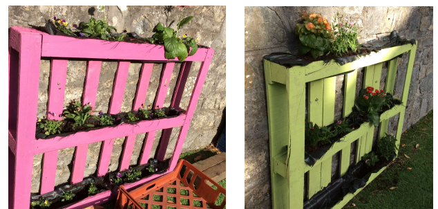
Figure 42: Living wall construction at Oldcastle Primary School
