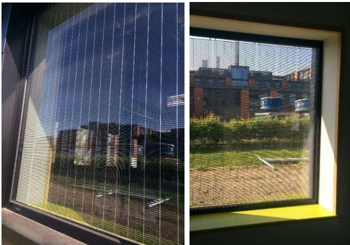
Figure 45 External (left) and internal (right) views of the PV window
