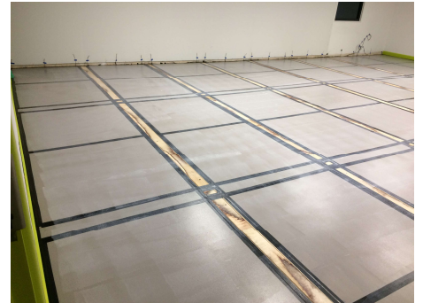
Figure 23: The heating panels installed
